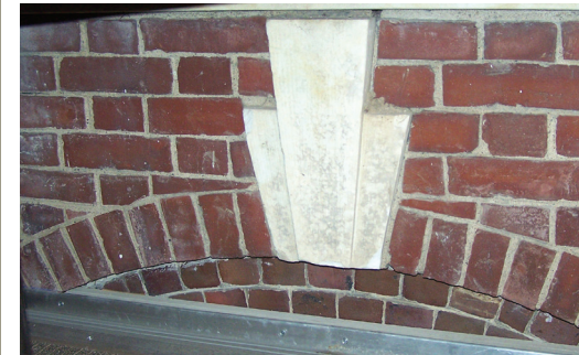
Window detail between old and new buildings.
